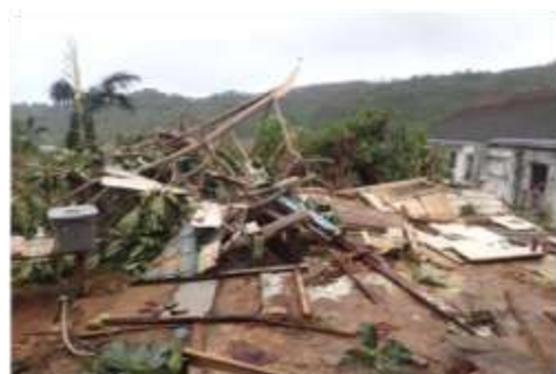
Typhoon Maysak left a wide path of destruction as many houses made of metal roofing or plywood sheets were blown over by strong gusts of wind.
